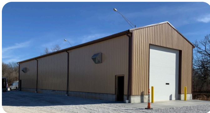
The new inspection building at Post D4 in Joplin, MO, is shown.
