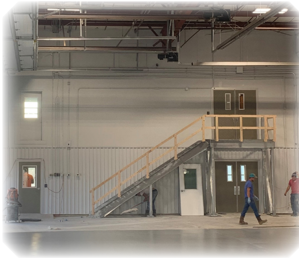
Workers complete the epoxy floor for the aircraft hangar on September 3, 2020.
