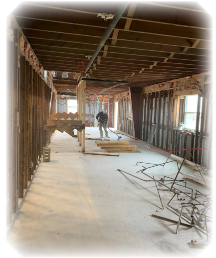
On May 12, 2020, workers completed the demolition phase.
