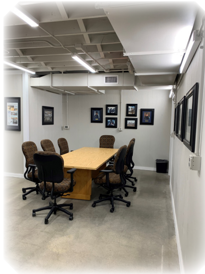
The new waiting area and conference room includes an exposed concrete floor and raised utilities.
